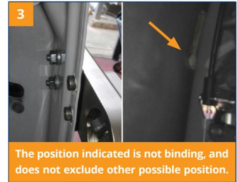
To fix the armor, in order to avoid the withdrawal (deformation) of the external sheet, it is advisable to interpose the counterplate and apply the nuts from the outside of the door (nuts on sight - see photo below).
